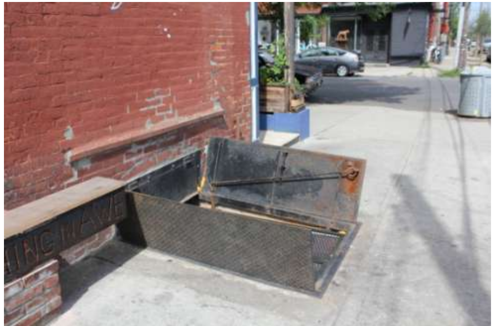
Sidewalk hatch door to basement
