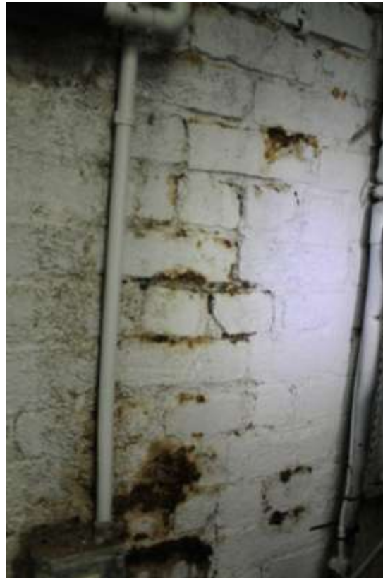
Ft. Defiance basement masonry wall
